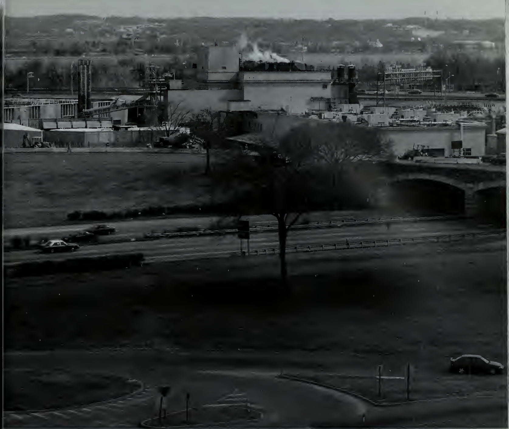
Heating and cooling plant
